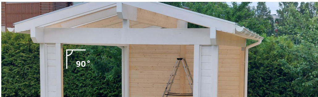
Figure 2. Make sure that the door openings are perpendicular
